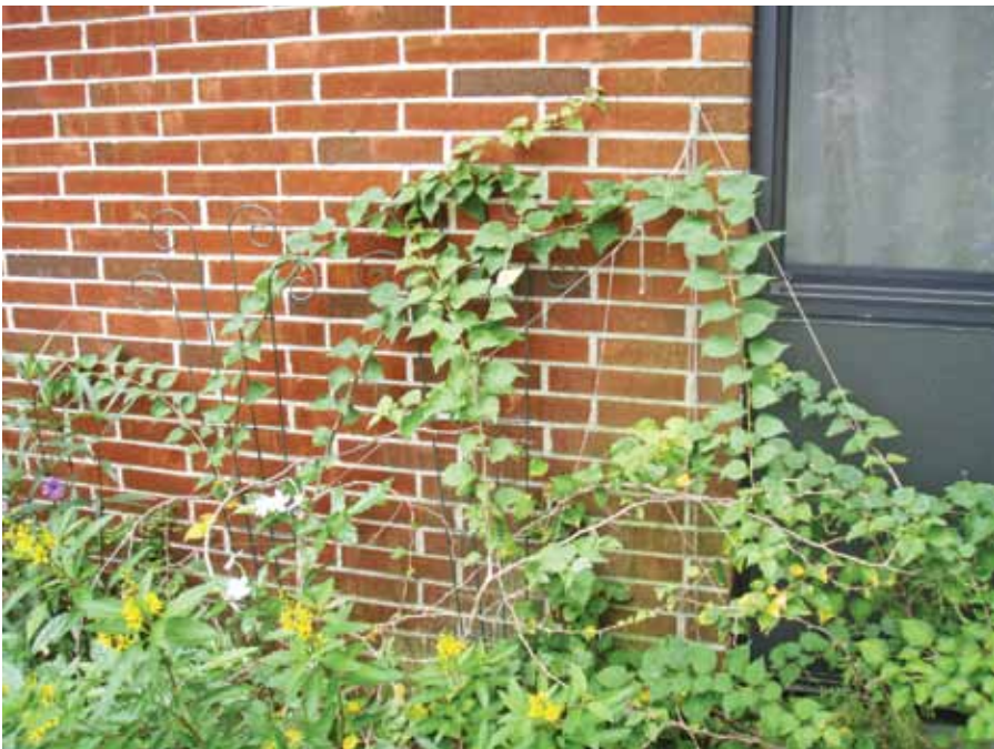
FIGURE 7 • Vining plants can give insects access into buildings.
